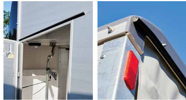
Protection from rain provided by the rain gutters above the doors and also in the rear area.
